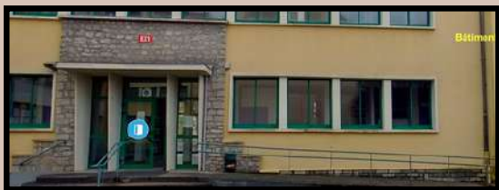
Ramps for people in wheelchairs
